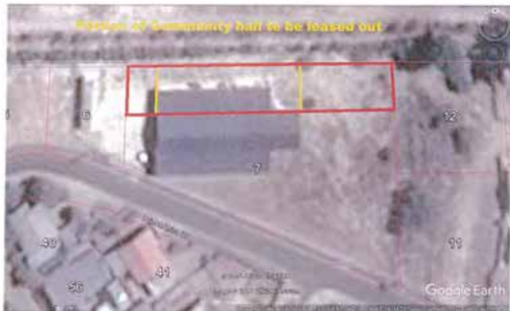
Fig 3: Portion of Community Hall
